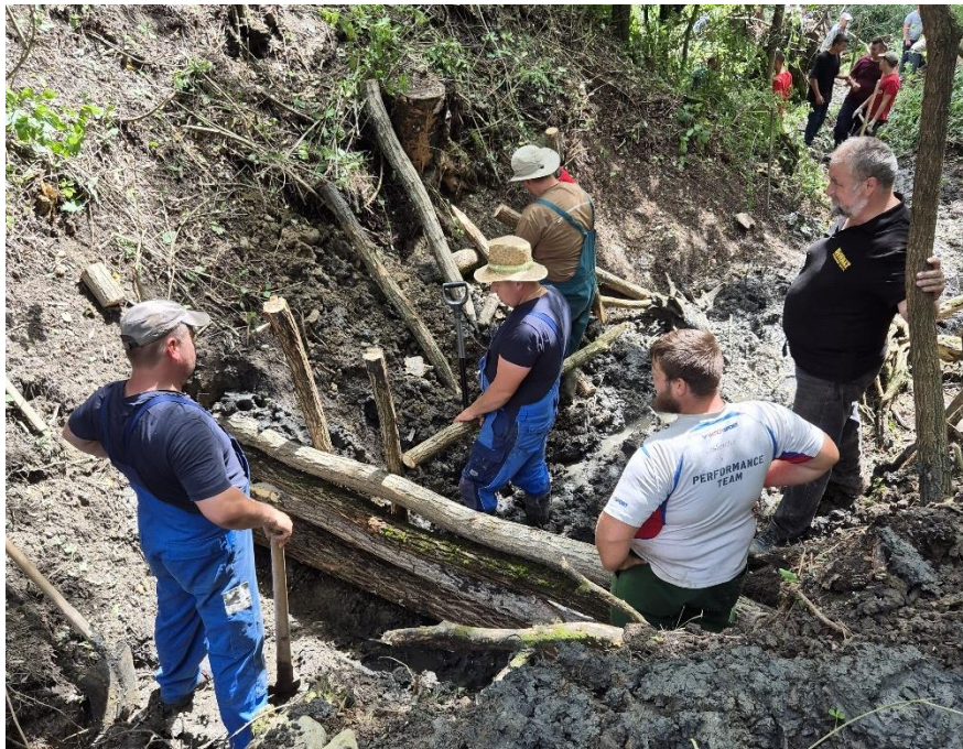
Photo: Community work to build weirs in Daia. Credit: Szilvia Bencze, ACNT
