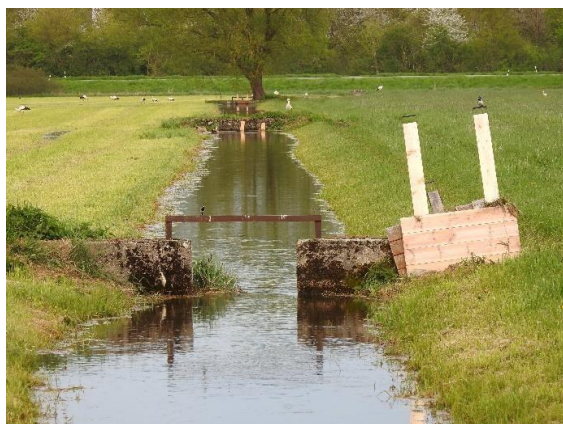
Photos: Various structures are used in the Queich River and in the ditches, such as simple sluice gates (top left), crank weirs (top right and bottom left), or a very large weir (bottom right - a fish ladder was built around this weir to ensure longitudinal connectivity. Photos: Peter Keller, Pirmin Hilsendegen
