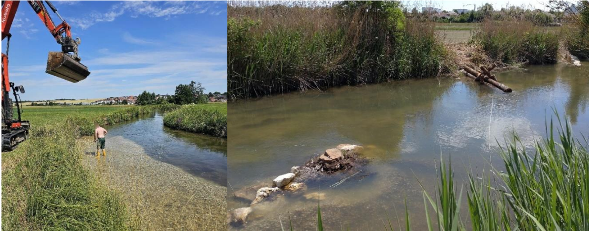
Photos 4 & 5: Installation of a gravel spawning ground for various river fish species and measures to improve flow dynamics through the placement of boulders, root-stocks and logs (Photo credit: Tobias Fuchs)
